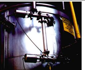
CyboCon CE (left) is mounted on the panel to replace PID and controls the tomato paste temperature. The holding tank (right) shows the 3-way valve that diverts the tomato paste back if its temperature is too high or too low.
